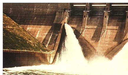
figura 1: Kinzua dam rehabilitation
